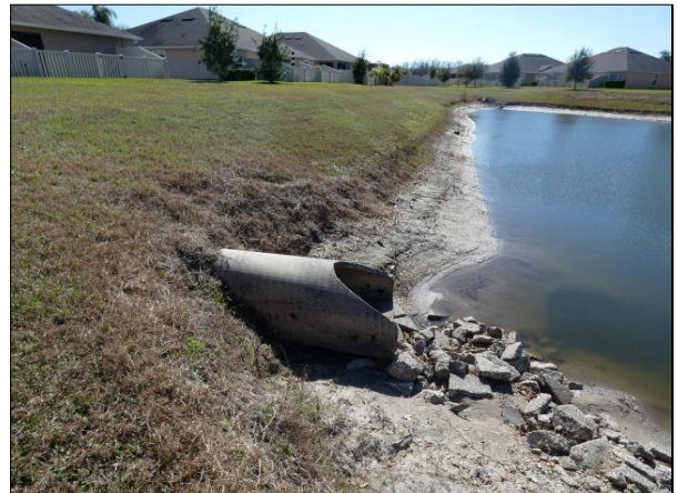
Stormwater Drainage Mitered End Section
