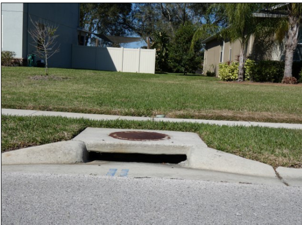
Stormwater Drainage Curb Inlet
